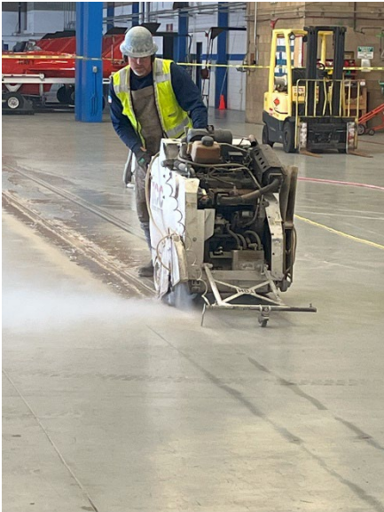
Cutting through existing concrete slab
