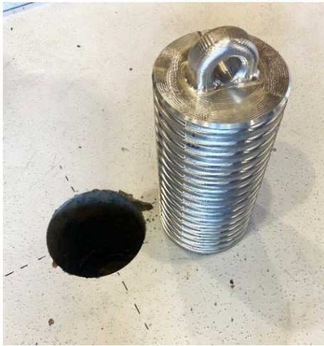
Figure 8-1: Concrete core drilled out of hangar slab to allow the ILDFA tie down point to be chemically anchored
