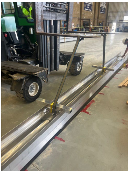
Place prefabricated aluminum trenches
