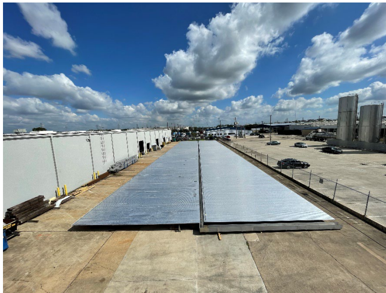
Figure 19-1: Flame detector testing was conducted on the ILDFA shown.
