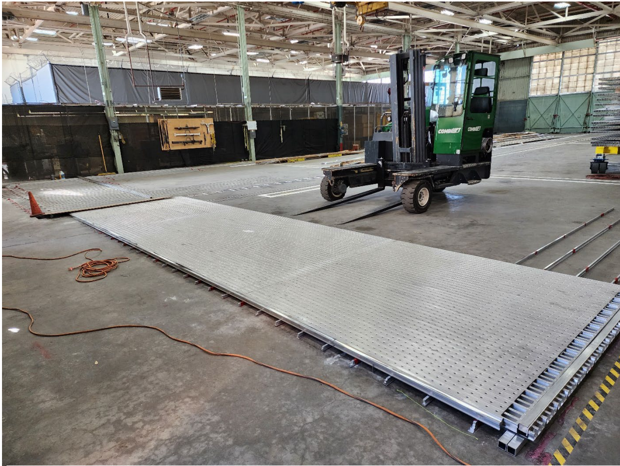
Figure 5-1: Aluminum flat bar used for shimming to proper slope requirements during installation
