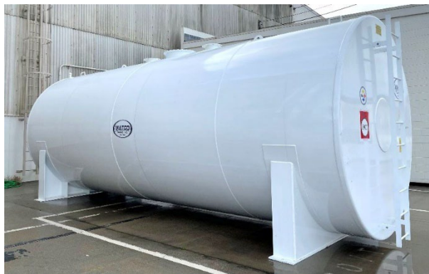
Figure 15-1: Example of 15,000 gallon (56,781 L) UL-142 steel aboveground tank; shown for reference only
