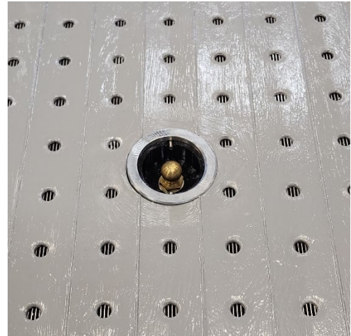
Figure 9-4: Grounding Point Inserted in ILDFA Floor Profile.
