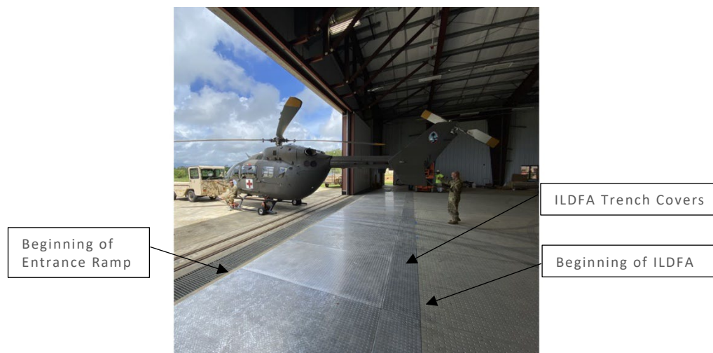
Figure 5-3: ILDFA with 1:48 sloped entrance ramp for helicopter with short elevation clearance
