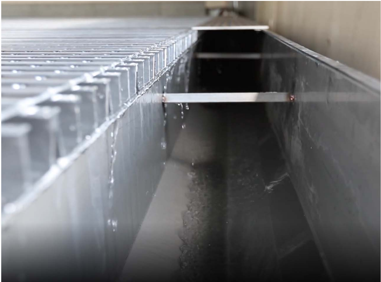
Figure 1-4: Trench shown with connection to floor profiles.
