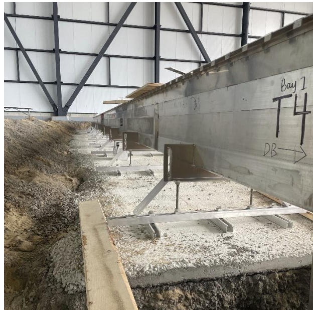
Figure 6-7: Step-by-step process of installing ILDFA prefabricated trenches
