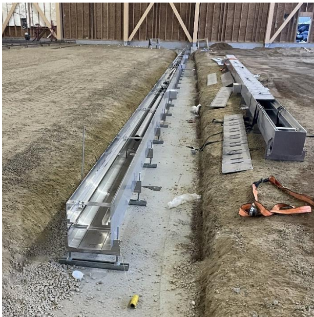
Figure 6-7: Step-by-step process of installing ILDFA prefabricated trenches
