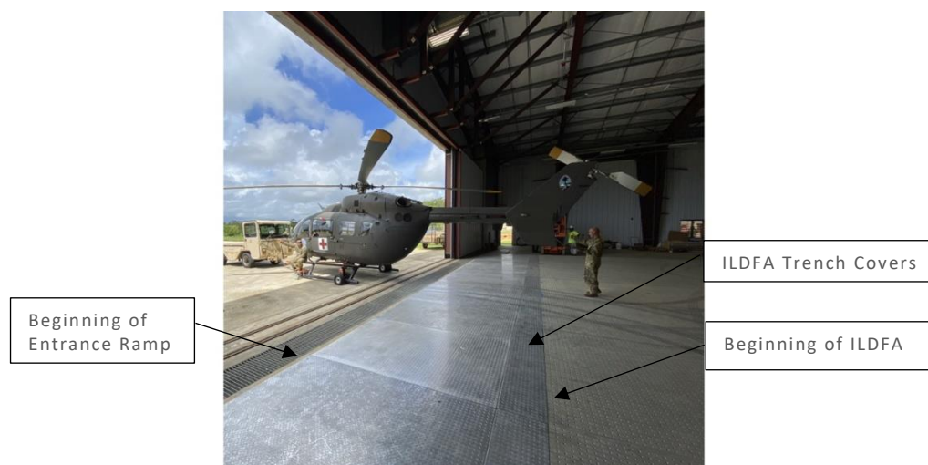
Figure 5-6: ILDFA with 1:48 sloped entrance ramp for helicopter with short elevation clearance
