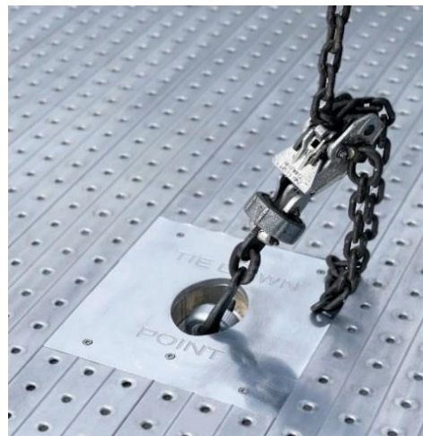
Figure 8-3: ILDFA tie down point example with aircraft chain connection
