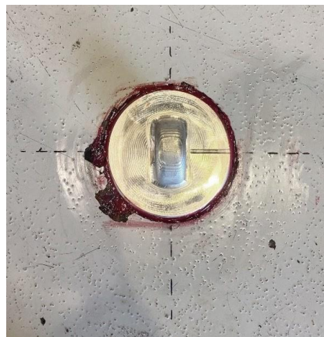
Figure 8-2: ILDFA tie down point chemically anchored into concrete slab
