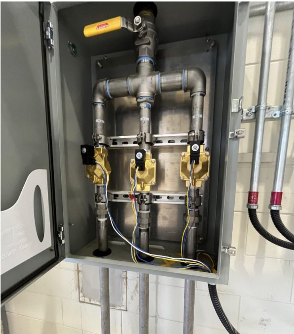
Solenoid Valves located outside of trench, housed in cabinet mounted on hangar wall.
