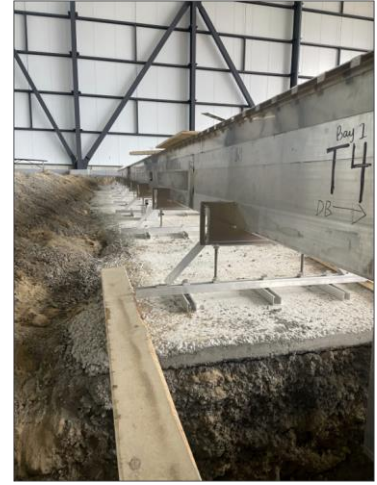
COLOCAR/ALINEAR ZANJA
